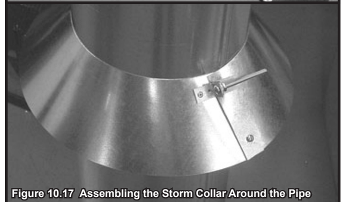
Figure 10.16 Assembling the Storm Collar
